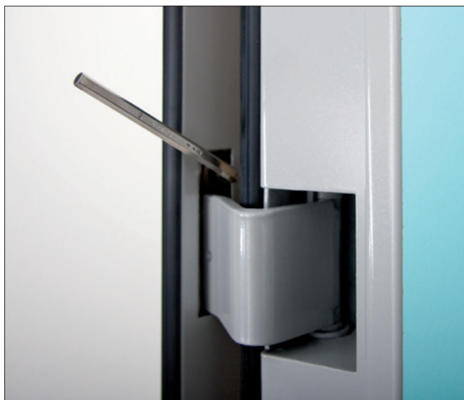
HIDDEN HINGES horizontal adjustment
