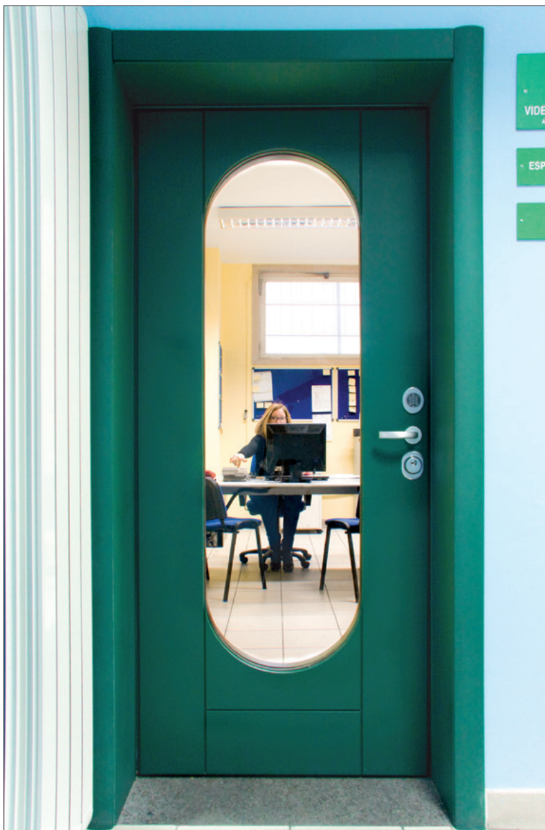
MOTORIZED LOCK Iseo x1R easy, with the possibility of remote opening (photo opening from the desk).
